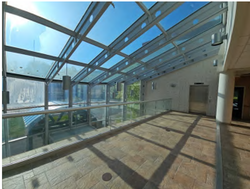
Figure 2 Main Lobby curtainwall system
